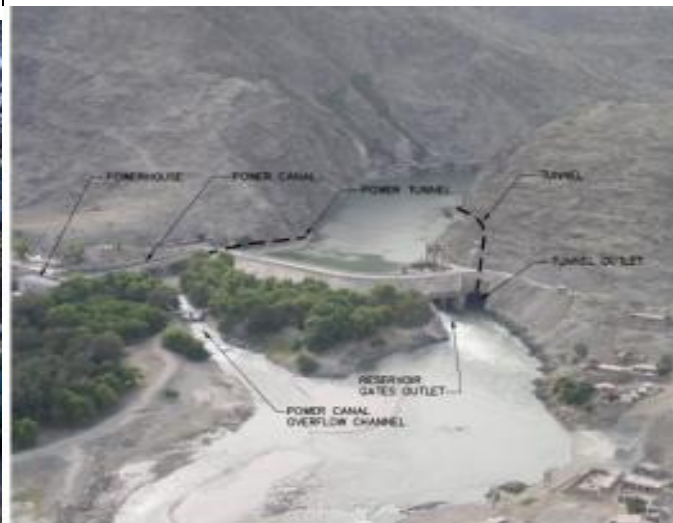
Front View of Darunta Dam
