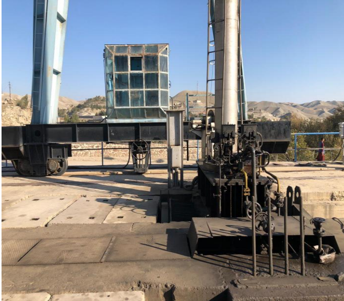
Figure 3: Spillway gate & crane view of Darunta dam
