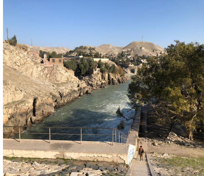
Figure 2: View of the downstream area
